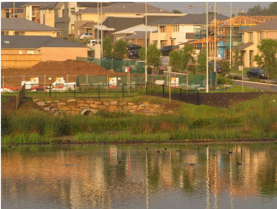
Figure 2.6.1. Constructed wetlands are becoming an increasingly common component of new residential developments to assist with stormwater storage and treatment as well as providing habitat for wildlife. (Photo: Cameron Webb, Medical Entomology, Pathology West – ICPMR Westmead.)
