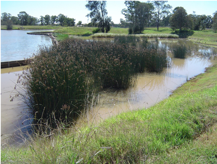
Figure 2.6.13. Structural barriers between the shallow macrophyte zones and deeper/open water components of wetlands will restrict the movement of aquatic plants but may reduce the impact of wind and wave disturbance, as well as movement of predators, into the macrophyte zone to reduce mosquito populations.
