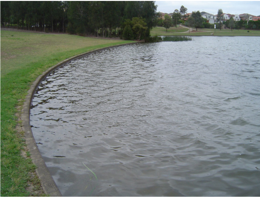
Figure 2.6.9. Wetlands that contain large areas of open water will not be suitable for mosquitoes due to disturbance from wind and wave action. A hard, vertical edge to the wetland further reduces the suitability of the habitats for mosquitoes. (Photo: Cameron Webb, Medical Entomology, Pathology West – ICPMR Westmead.)
