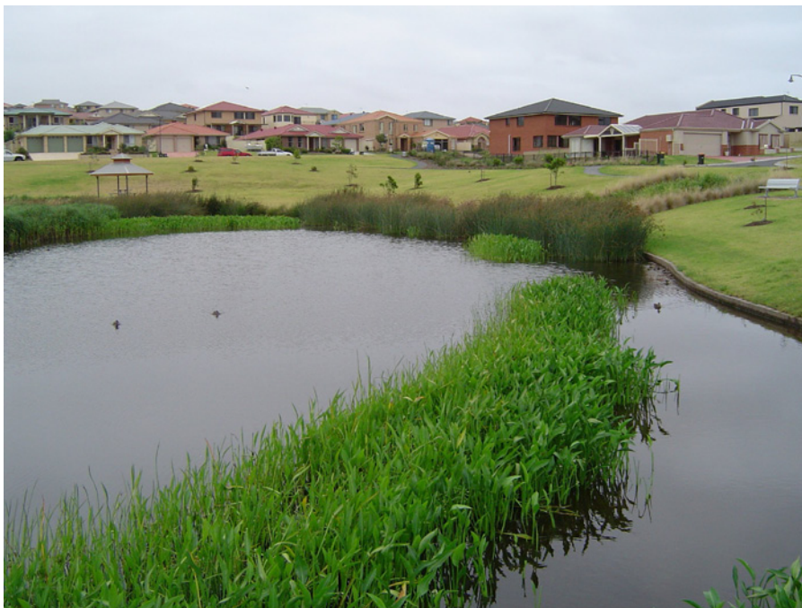
Figure 2.6.12. The suitability of macrophyte zones for mosquitoes can be reduced by locating the vegetated shallow water areas away from the wetlands edge. In addition, the inclusion of a hard vertical edge around the wetland margins further reduces the suitability of mosquitoes in the macrophyte zone by increasing access of predatory fish and other macroinvertebrates. (Photo: Cameron Webb, Medical Entomology, Pathology West – ICPMR Westmead.)
