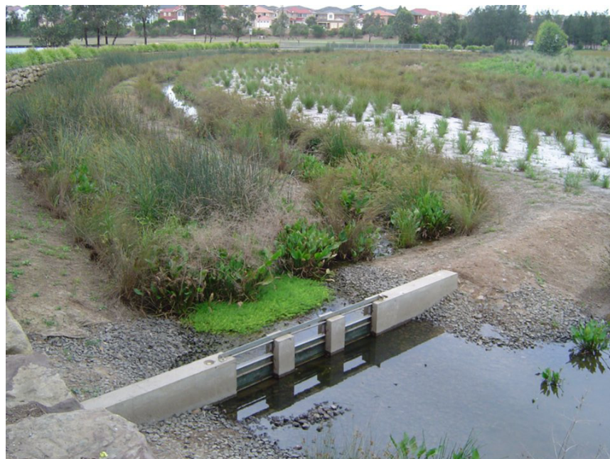
Figure 2.6.10. The mosquito important habitats for mosquitoes within a constructed wetland are the shallow, well vegetated macrophyte zones. These habitats can vary substantially depending on the design of the wetland and abundance and diversity of aquatic vegetation. (Photo: Cameron Webb, Medical Entomology, Pathology West – ICPMR Westmead.)
