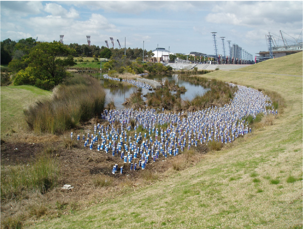
Figure 5.1.1. Northern Water Feature, a water quality management wetland in Sydney Olympic Park.
